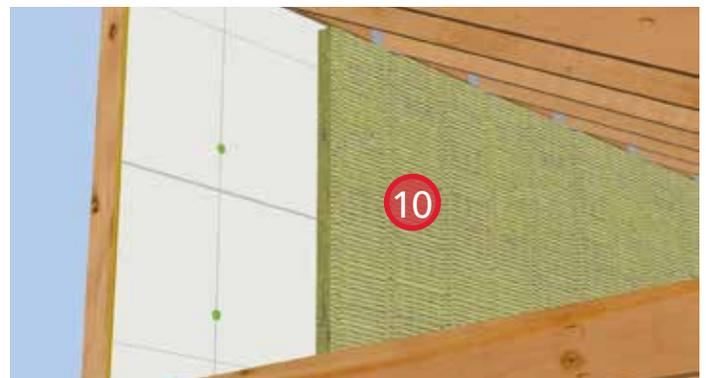
10. Install ROCKWOOL COMFORTBOARD™ on the exterior of the wall between canopy ledger boards with recommended fasteners.
