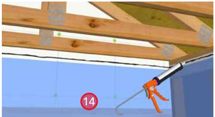
14. Install a bead of acoustical sealant along the sheathing membrane in line with the lower top plate of the exterior wall.
