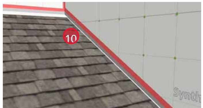
10. Seal all edges of the sheathing membrane with sheathing tape.
