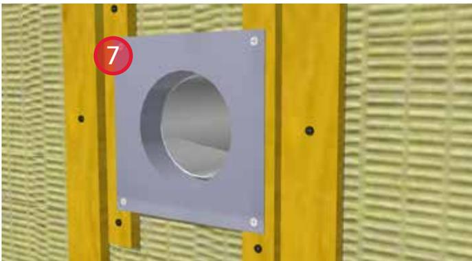
7. Install adaptor flange and secure to the support strapping.
