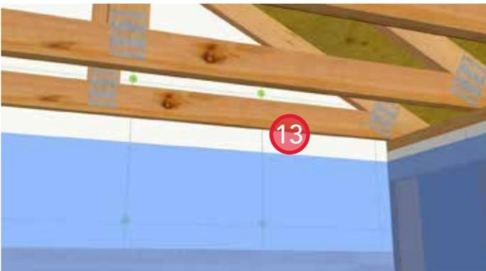
13. Install poly on the walls and fasten to the sheathing membrane with staples.
