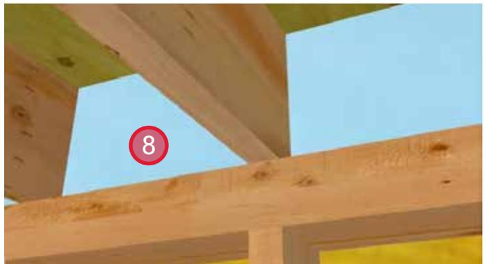
8. Install rigid insulation on the interior of the rim joist. ROCKWOOL COMFORTBOARD™ and ROCKWOOL COMFORTBATT® can be used to meet thermal barrier requirements for foamed plastics.
