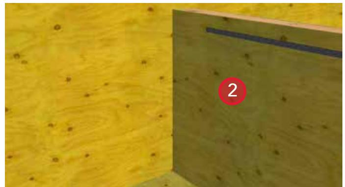
2. Frame the vented guard wall and slide into place over the first stud.
