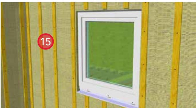
15. Install ROCKWOOL COMFORTBOARD™ at the window head and secure with strapping. Provide bugscreens at the top and bottom of the strapping.
