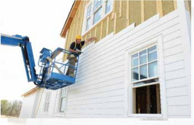
Generally, the water shedding surface (WSS) is the outer surface of the wall assembly and is designed to manage bulk water in the system. A rainscreen approach assumes that some incidental moisture will likely penetrate behind the WSS and must be allowed to drain through the rainscreen cavity and out of the assembly at cross-cavity flashing locations. Water removal in the ventilated wall cavity also occurs through evaporation and is facilitated by ventilation.
