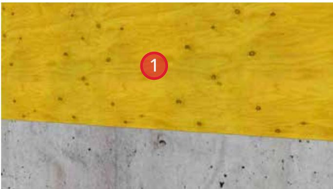
1. Typical wood frame construction at sheathing installation stage. Install wood framing on concrete curb extending 8" above concrete deck.
