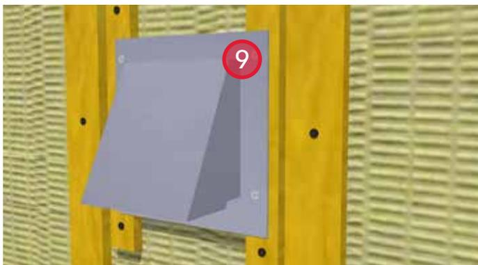
9. Install exhaust vent hood, bedded in sealant to the adaptor flange.
