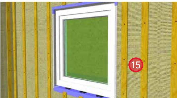
15. Install ROCKWOOL COMFORTBOARD™ and secure with strapping. Provide bugscreens at the top and bottom of the strapping.
