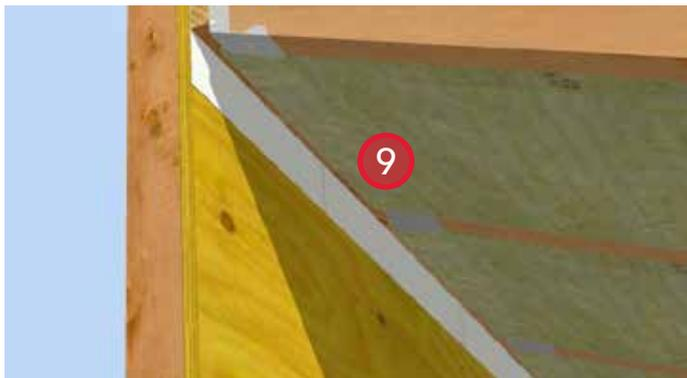
9. Install ROCKWOOL COMFORTBATT® in the rafter cavities.
