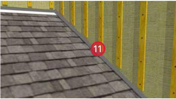
11. Install ROCKWOOL COMFORTBOARD™ and secure in place with strapping. Provide bugscreens at the top and bottom of the strapping.
