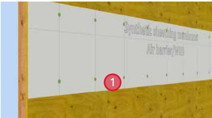
1. Install a starter strip of sheathing membrane to extend above and below the roof plane. This will allow for air-barrier transition to be completed later.
