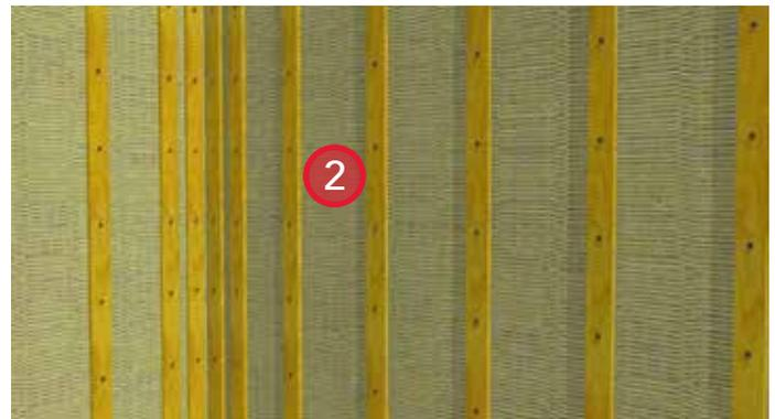
2. Install ROCKWOOL COMFORTBOARD™. Use strapping to secure the insulation in place with recommended fasteners. Provide bugscreens at the top and bottom of the strapping.
