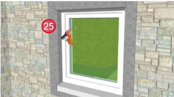
19. Apply sealant around the perimeter of the window (top and sides) between the frame and the cultured stone trim.
