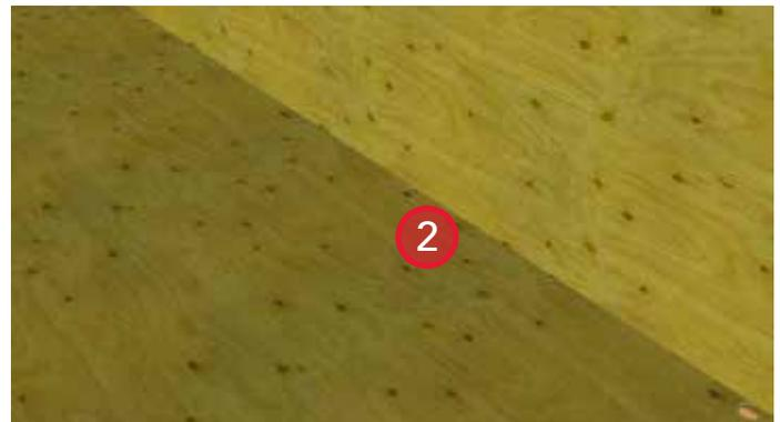
2. Provide ventilation in the roof deck. Drill 1" diameter holes along the perimeter. Roof ventilation will likely be supplemented with dog house vents.
