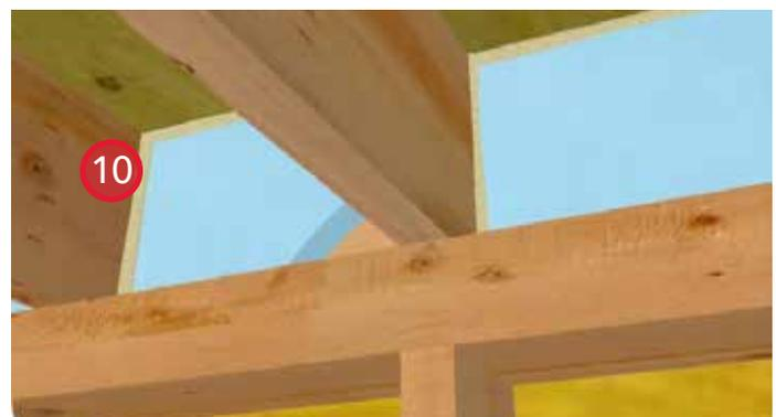
10. Install spray foam around the perimeter of the joist bay, sealing to the rigid insulation, top plate, joists and subfloor for air tightness and thermal barrier continuity.
