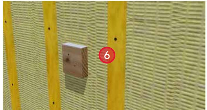
6. Install ROCKWOOL COMFORTBOARD™ and strapping. Provide bugscreens at the top and bottom of the strapping.
