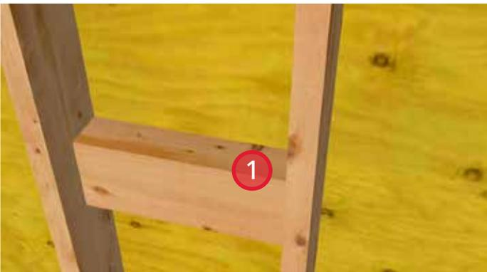
1. Install two blocks between interior studs where railing penetration will occur. This will provide structural support for the engineered railing attachment.
