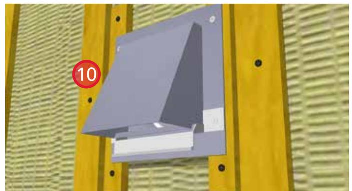
10. Install prefinished metal flashing below the exhaust vent hood.
