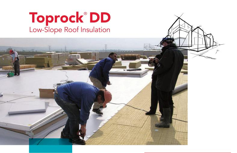
ROCKWOOL Toprock<sup>®</sup> DD is a rigid and high-density, uncoated stone wool insulation board for low-slope roof applications. Toprock DD is a suitable substrate for mechanically-attached membrane systems in low slope roofing.
