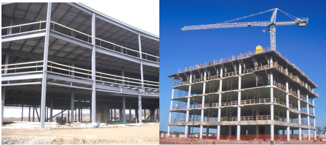
Figure 2: Steel Framed (left) and Concrete Framed (right) superstructure systems
