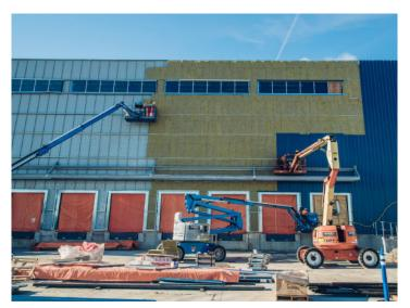
When exposed to clement weather conditions, ROCKWOOL unfaced exterior wall insulation products, when installed vertically, may remain exposed for up to 90 days without negatively affecting their properties. Faced insulation product Cavityrock<sup>®</sup> Black, may be exposed for up to 30 days without adverse effects.
