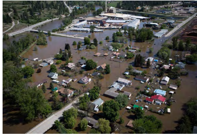
→ Flooding hits Grand Forks, British Columbia and the local ROCKWOOL manufacturing site.
