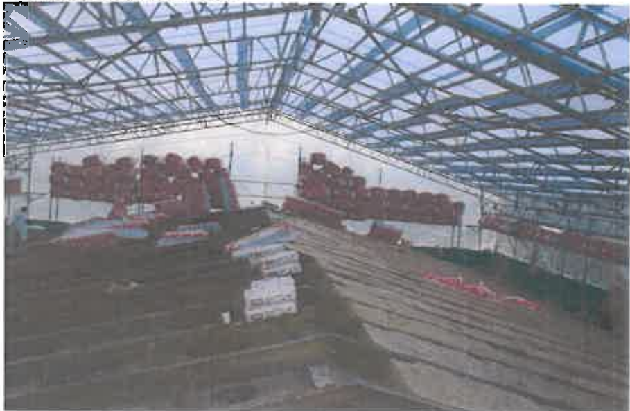
Photo no. 4, The construction site
