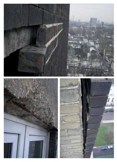
Figure 8: Brickwork in a state of disrepair and exposed concrete
