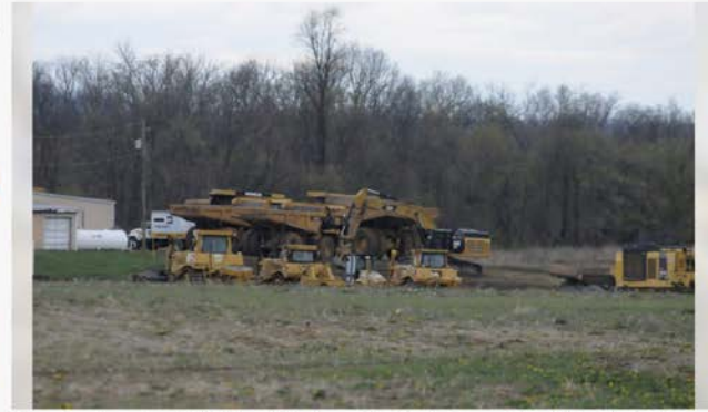
Heavy earth moving equipment at the Rockwool site in Kearneysville Wednesday afternoon. (Journal Photo by Ron Agnir)
