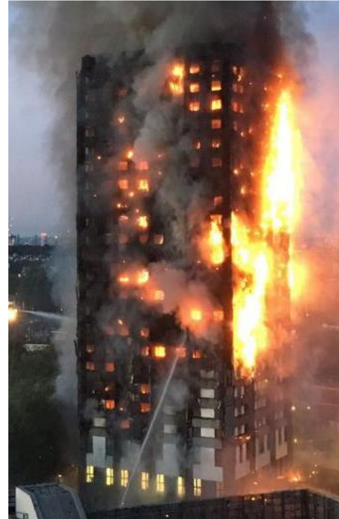
Grenfell Tower, London (2017)
