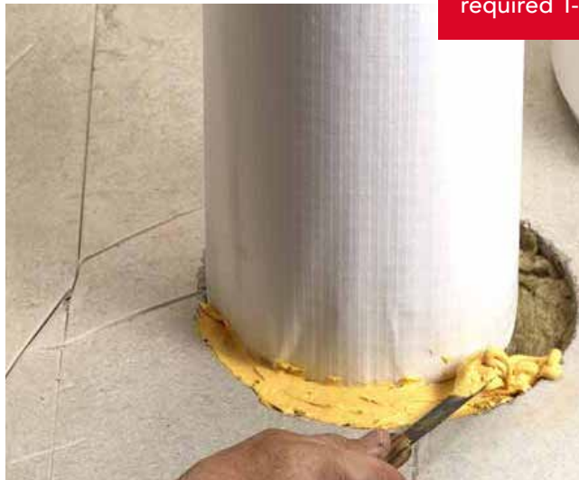
Stone wool insulation installed in annular space of rated floor assembly
