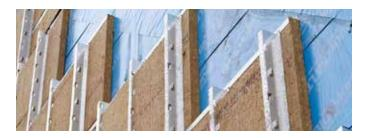
Crossing Z-girt cladding support system with custom punched vertical Z-girt profiles used to retain ROCKWOOL CAVITYROCK  $^{\!\!\circ}$  insulation.
