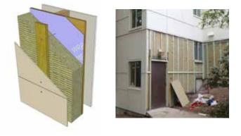
Long screws through vertical wood strapping and rigid ROCKWOOL COMFORTBOARD<sup>™</sup> insulation on a multi-family residential project.
