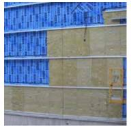
Horizontal Z-girts over a steel stud wall assembly. Girts are fastened every 36" here to reduce the thermal bridging.
