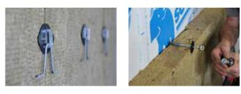
Examples of masonry ties installed through ROCKWOOL CAVITYROCK  $^{\circ}$  insulation.
