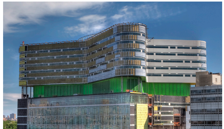
Figure 2: Exposed Cavityrock® during construction of RUSH University Medical Center in Chicago, IL
