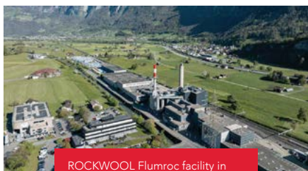
ROCKWOOL Flumroc facility in Switzerland
