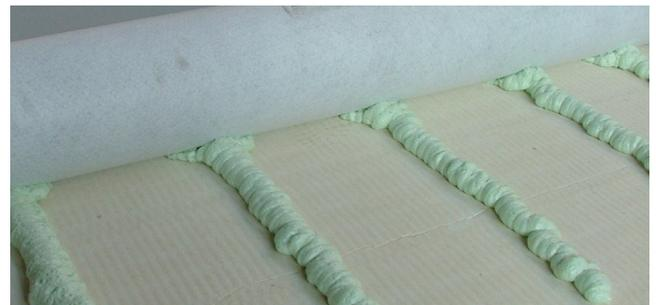
A bonded membrane incorporating HardRock Multi-Fix (DD)
