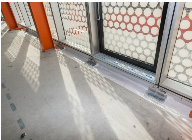
SoftSeal System installed as a linear joint seal
