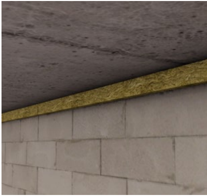
Figure 1 Linear FireStop 2A
