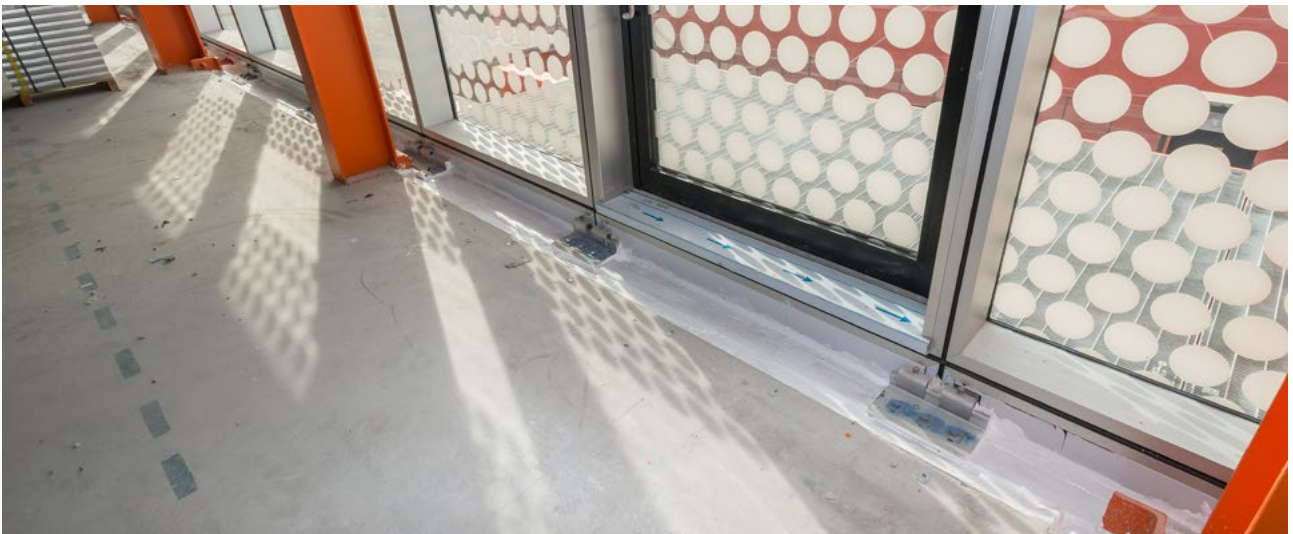
SoftSeal installed as a linear joint seal
