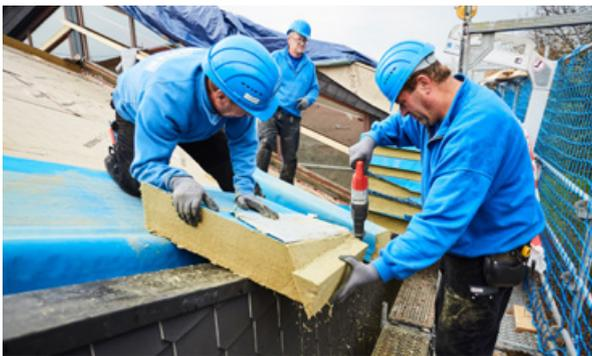
When it came to insulation, the team at Kühne GmbH from Kassel laid non-combustible and pressure-resistant stone wool panels from ROCKWOOL.
