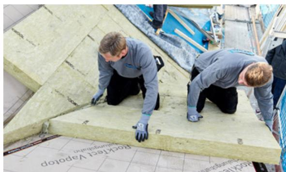
A ROCKWOOL weatherproof vapour barrier was installed to ensure the roof was initially protected, followed by the ROCKWOOL fire-safe insulation solution for pitched roofs.
