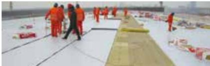
Flexible waterproof membrane roof system
