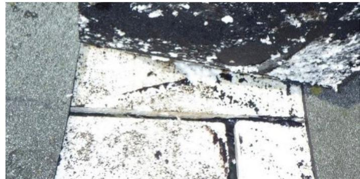
**Figure 2** Permanent shrinkage of EPS insulation in a conventional roof assembly, potentially due to high in-service temperature or initial application into hot asphalt adhesive.
