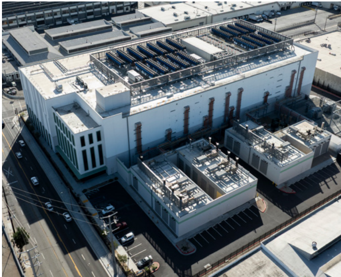
Figure 14: Aerial View of On-site Power Generation Systems Adjacent to the Data Center
