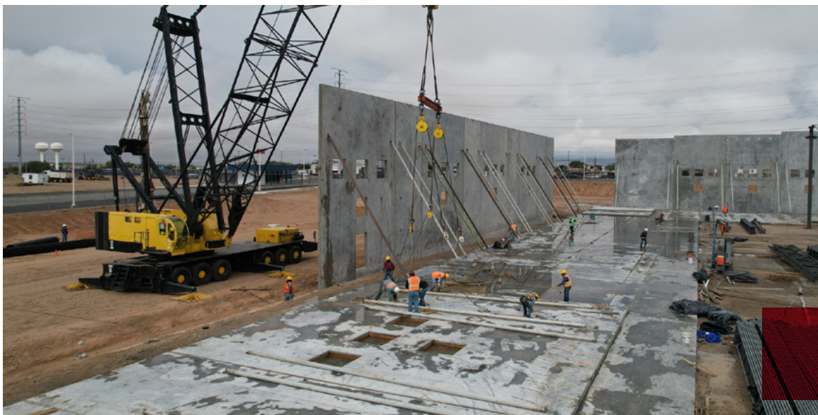
Figure 4: Tilt-up panel erection: site-cast concrete wall panels cast horizontally, lifted into position to form the building enclosure.
