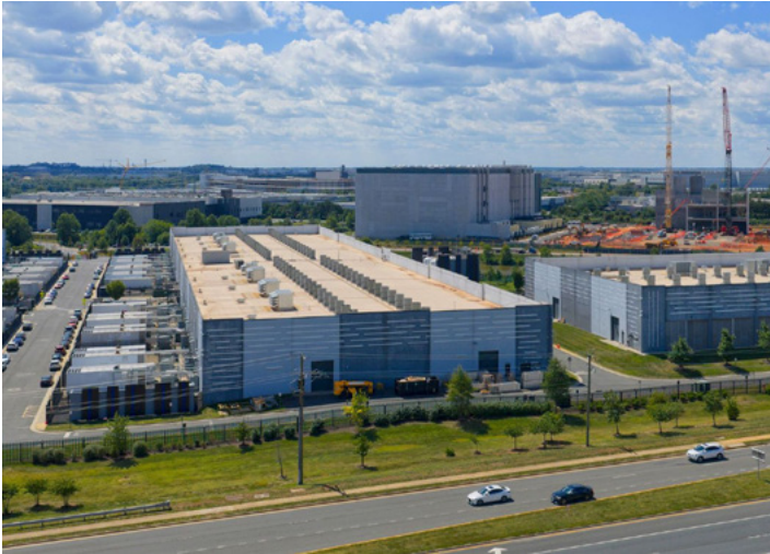
Figure 9: Aerial view of data centers in Ashburn, Virginia
