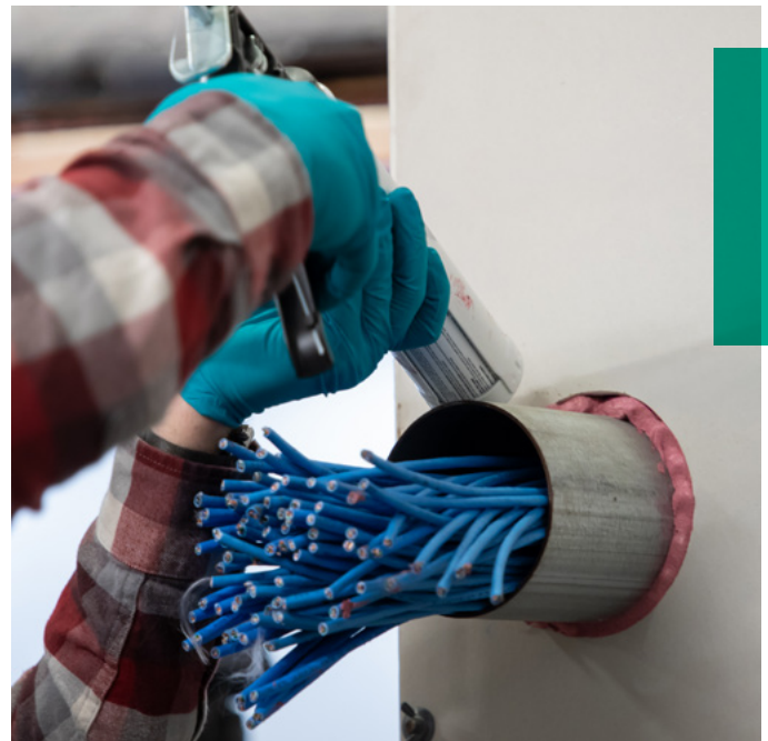
Figure 3: A mineral wool forming material is commonly installed within penetration openings and then sealed with a compatible fire-stop caulk.
