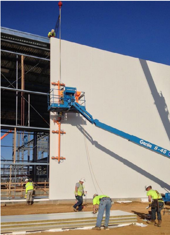
Figure 7: Installation of insulated metal panels (IMPs) with a non-combustible stone wool core: factory-fabricated panels provide integrated air, vapor, water, and thermal barriers, enabling rapid on-site erection while enhancing passive fire resistance.
