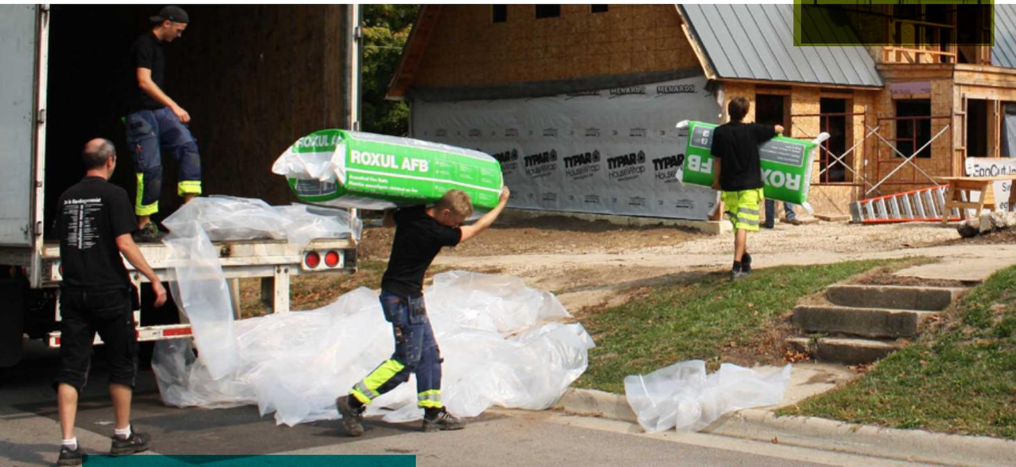
Layering. That is the key to the Scandinavian principle of residential construction. The idea that layering insulation in different stages within the wall assembly eliminates thermal bridging and creates an energy efficient, continuously insulated, air-tight envelope has been part of building practices in Sweden and other parts of Scandinavia for years.
