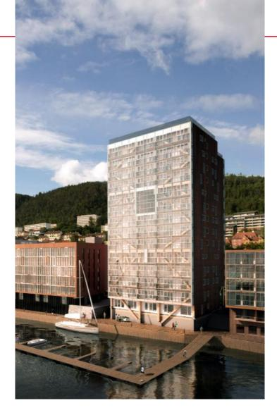
The world's tallest wooden house "Treet" in Bergen, Norway with ROCKWOOL facade insulation contributing to the apartments being built according to passive house requirement
