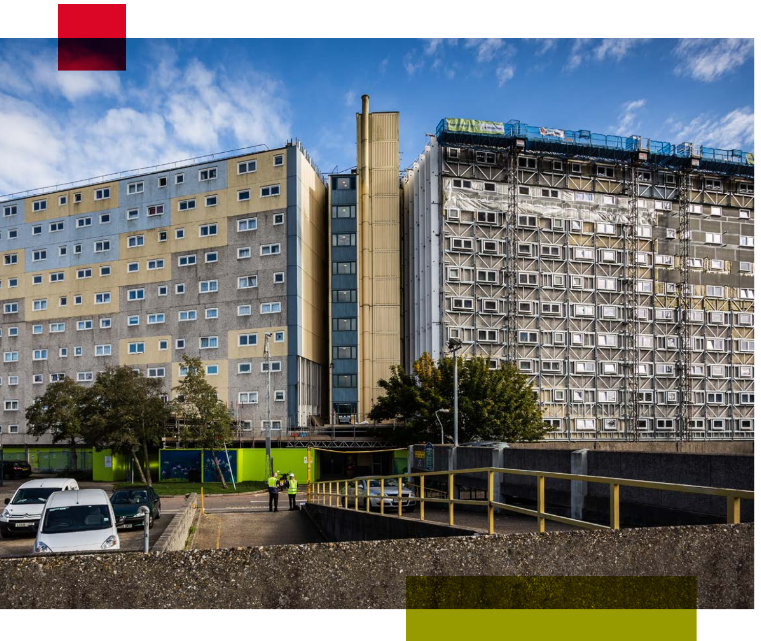
Wilmcote House - during renovation. Source: ROCKWOOL
