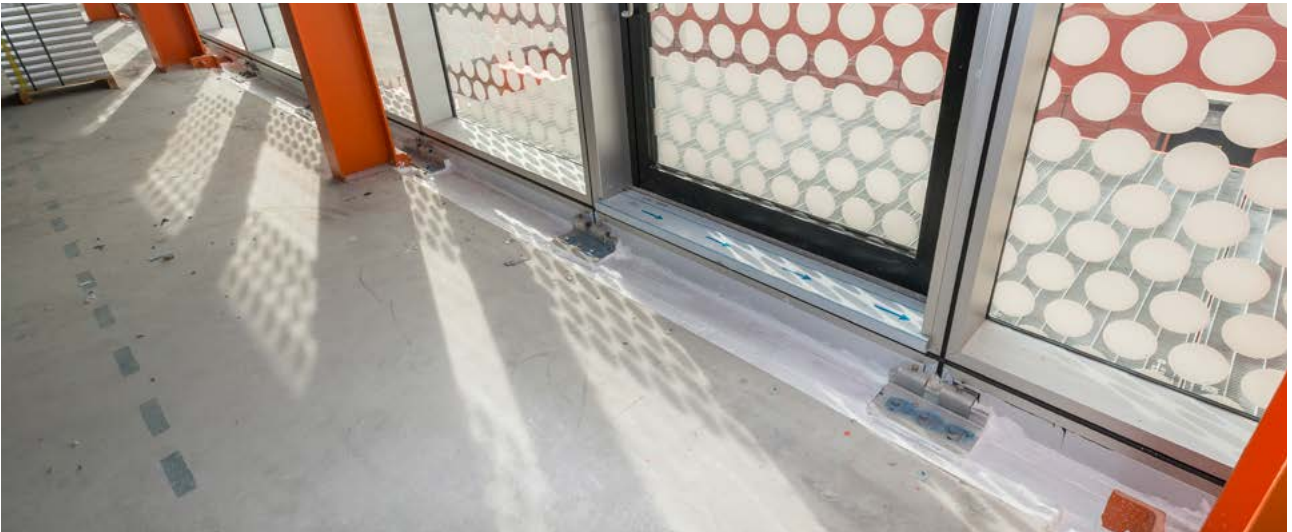
SoftSeal installed as a linear joint seal
